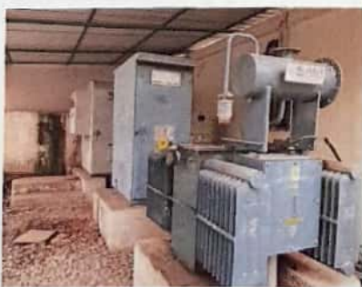
TRANSFORMER RATING 200 KVA
