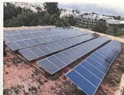
ROOF TOP SOLAR SYSTEM 160 KWp
